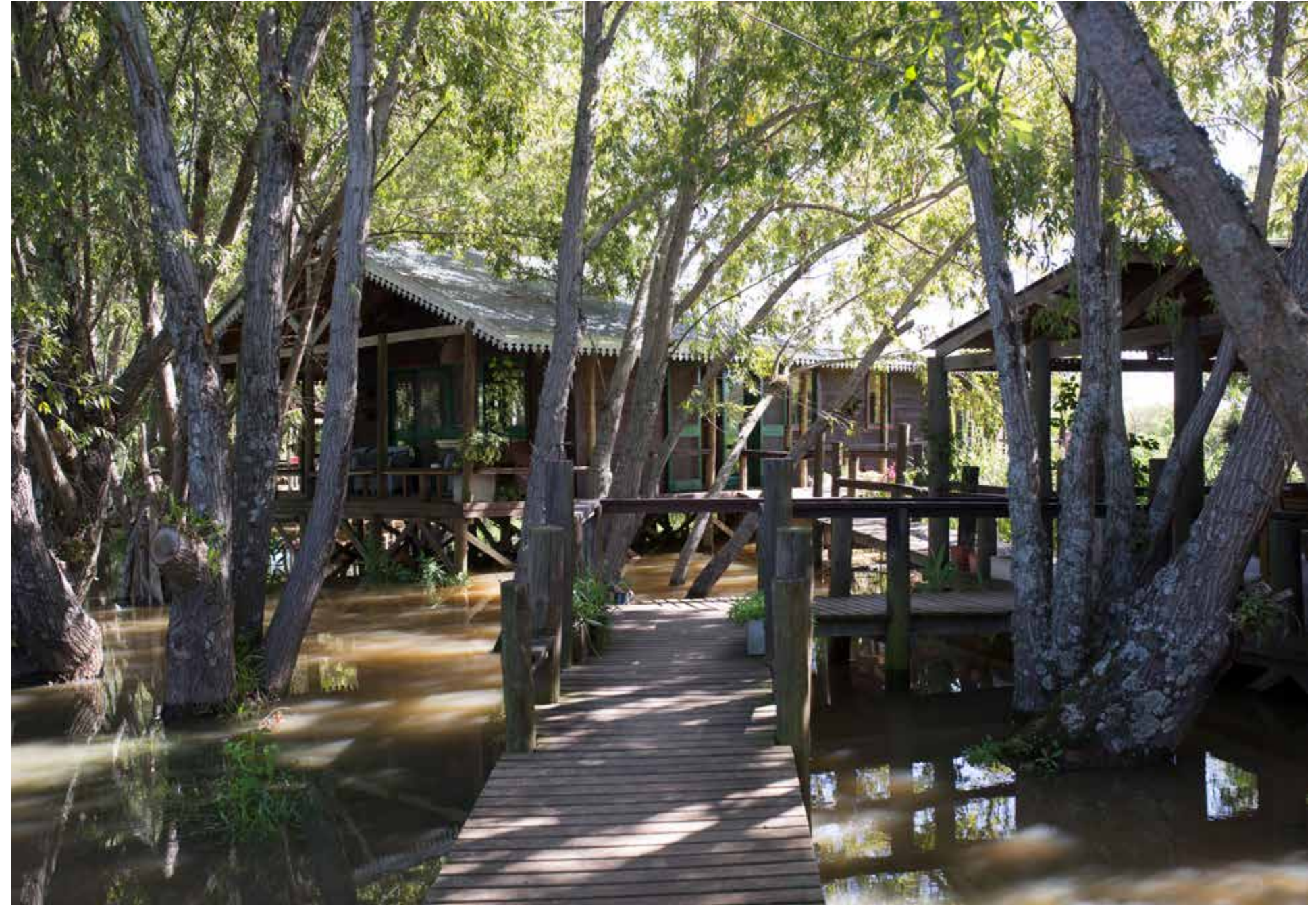
Perched above the Delta floor, the lodge is nestled amidst the low canopy and reeds. Constructed in the traditional Delta style, it features local hardwood and stands gracefully on stilts above the water.
